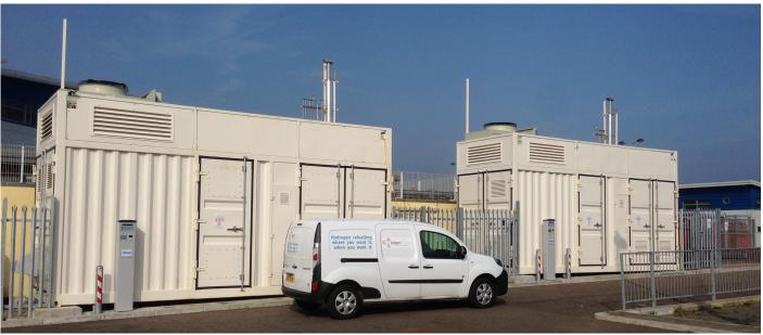
H2Tec's H2Key Gen is a self-contained, fully integrated hydrogen refuelling station for hydrogen vehicles. In its full format it generates hydrogen from local water and electricity supplies, and compresses, stores and dispenses it to provide an autonomous transport refuelling system.
